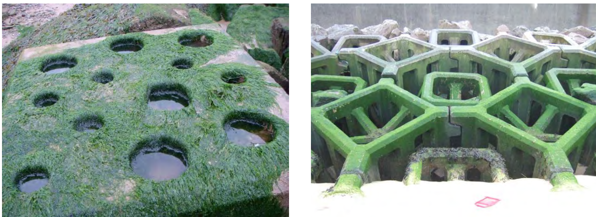
Figure 9 – Precast Cisterns & Wave Absorbing Structures, Colwyn Bay & North Wirral
